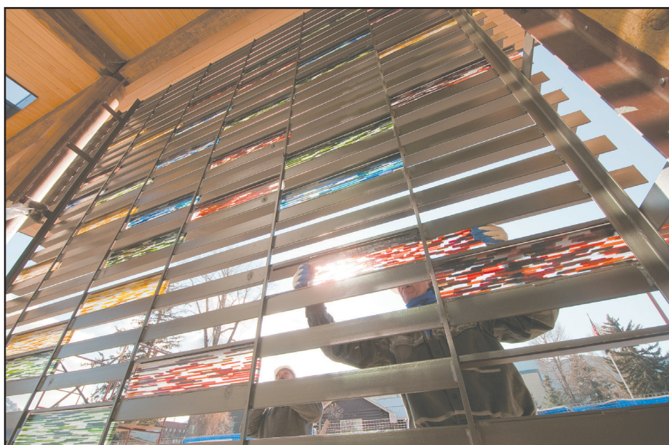
David Anderson of Jackson Paint and Glass affixes a piece of Frechette's work on Nov. 7. The buildings's sunscreens were modified to accommodate the art.
